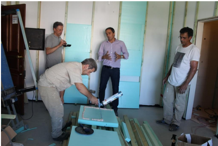
Figure 8: A moment during the renovation of the nZEBoffice+.
