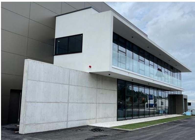
Figure 1: Danosa headquarters in Portugal, east façade.
