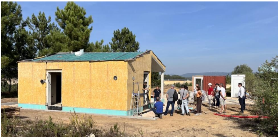
Figure 3: A practical workshop during the construction phase.
