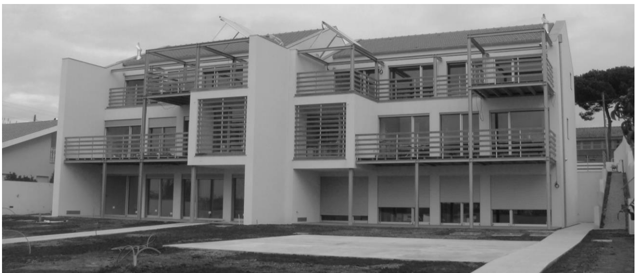
Figure 1: Exterior view of the first Passive Houses in Portugal
